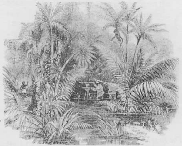
Surveying original alinement of the Panama Railroad in the jungle swamp. (Clifton E. Hull collection)
