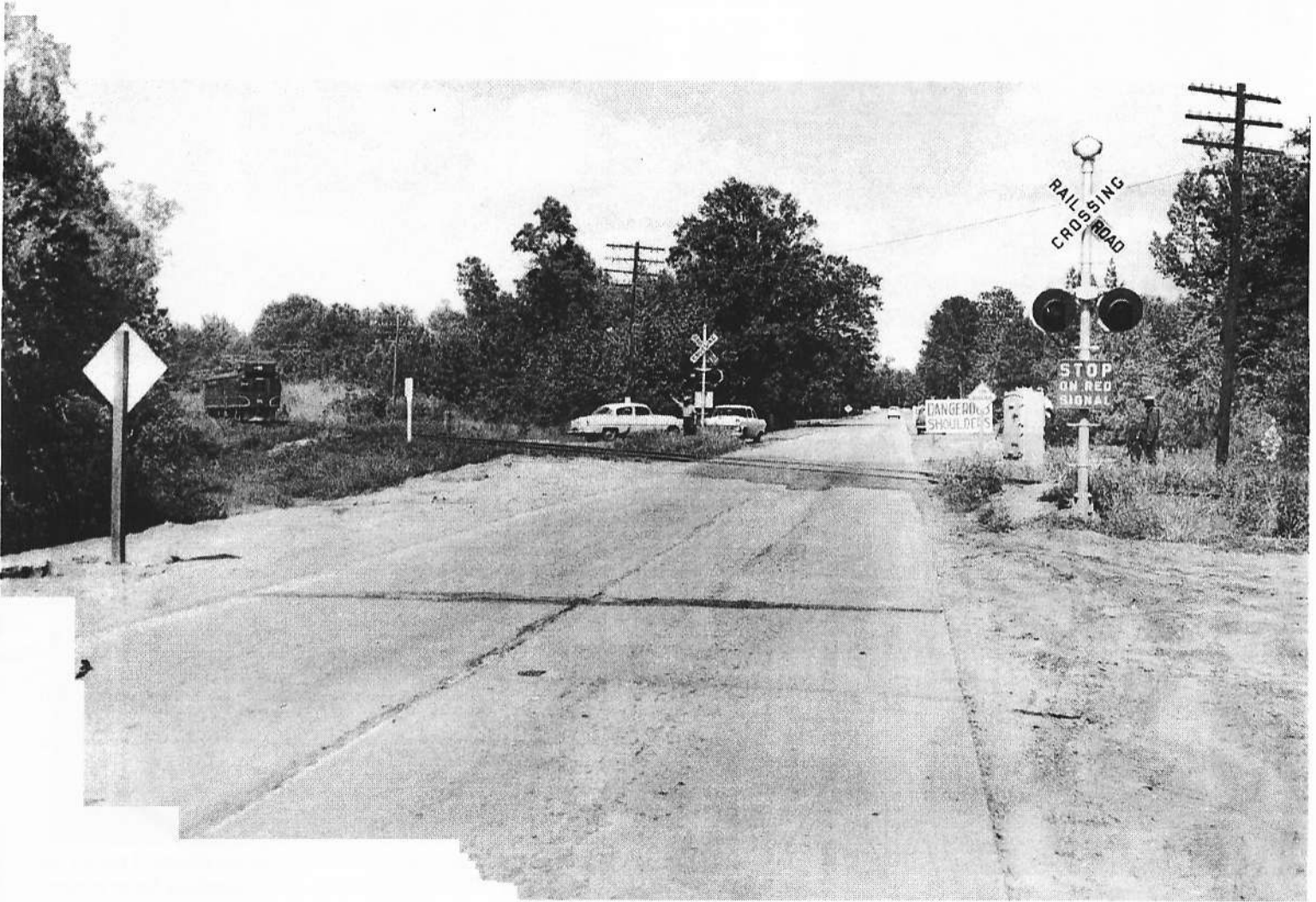
A Rock Island accident investigation photo taken at the Highway 167 crossing near Clay, Louisiana between 2 and 3 p.m. May 10, 1957 in connection with a fatality at the grade crossing on May 7. Notice southbound Rock Island Passenger Train #31 approaching the crossing from north end (left) at a point 250 feet north of crossing. (L. T. Walker collection)
