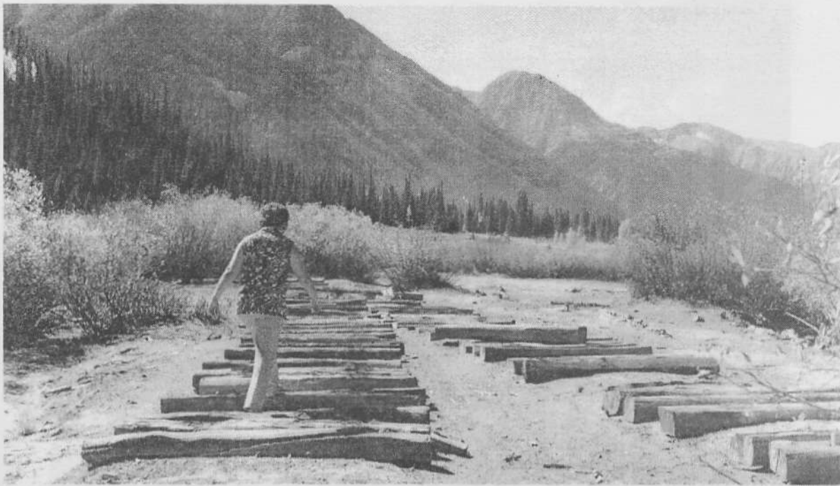
Some of these rough hand-hewn crosssties were laid in 1896 to form a balloon turnaround for reversing narrow gauge engines on the Silverton Northern Railroad near Eureka, Colorado. (Gene Hull photo)
