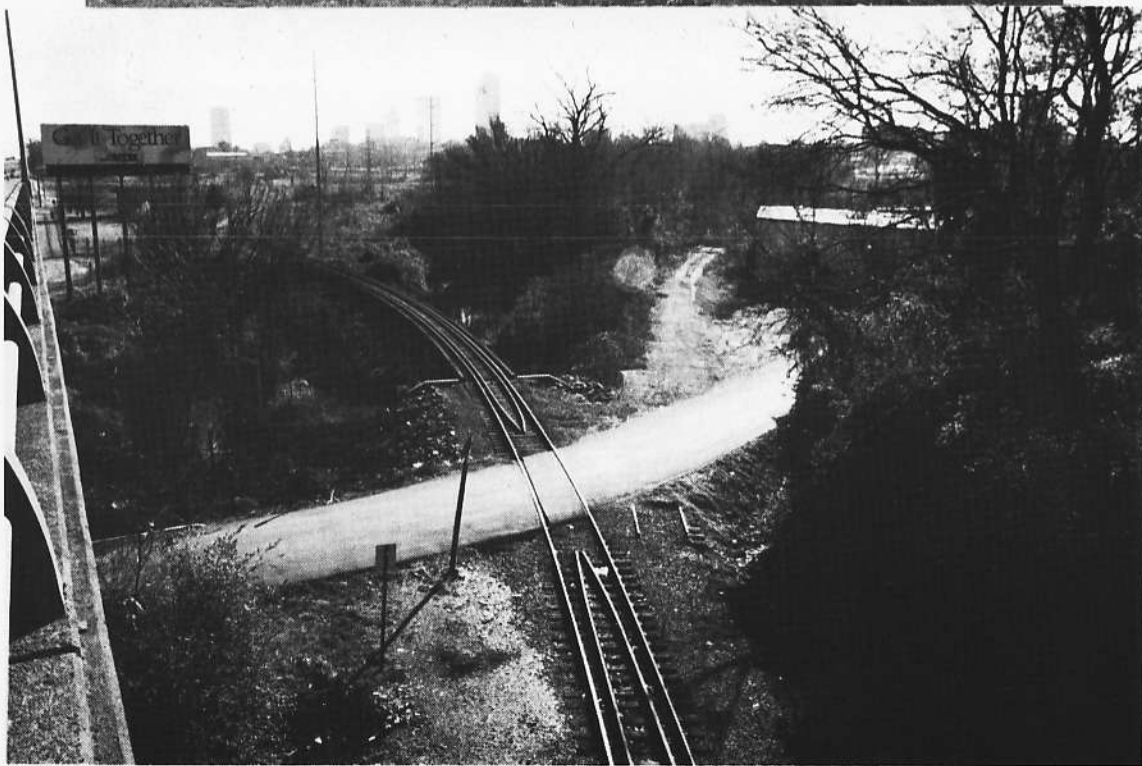
TOP - Missouri & North Arkansas depot, now used as a residence, in Bellefonte, Arkansas on October 29, 1988 looking at the south end. ( Bernie Harville, Jr collection ). BOTTOM - Little Rock & Western RR is building a line on a "new" grade, which will connect with the Union Pacific in front of Union Station in Little Rock (a half mile or so past the trees in the center). This "new" grade happens to be on the exact right of way the old Rock Island Sunbelt Route used. The route currently used was bought and will be used for office buildings. ( John Jones photo, late December 1997 )
