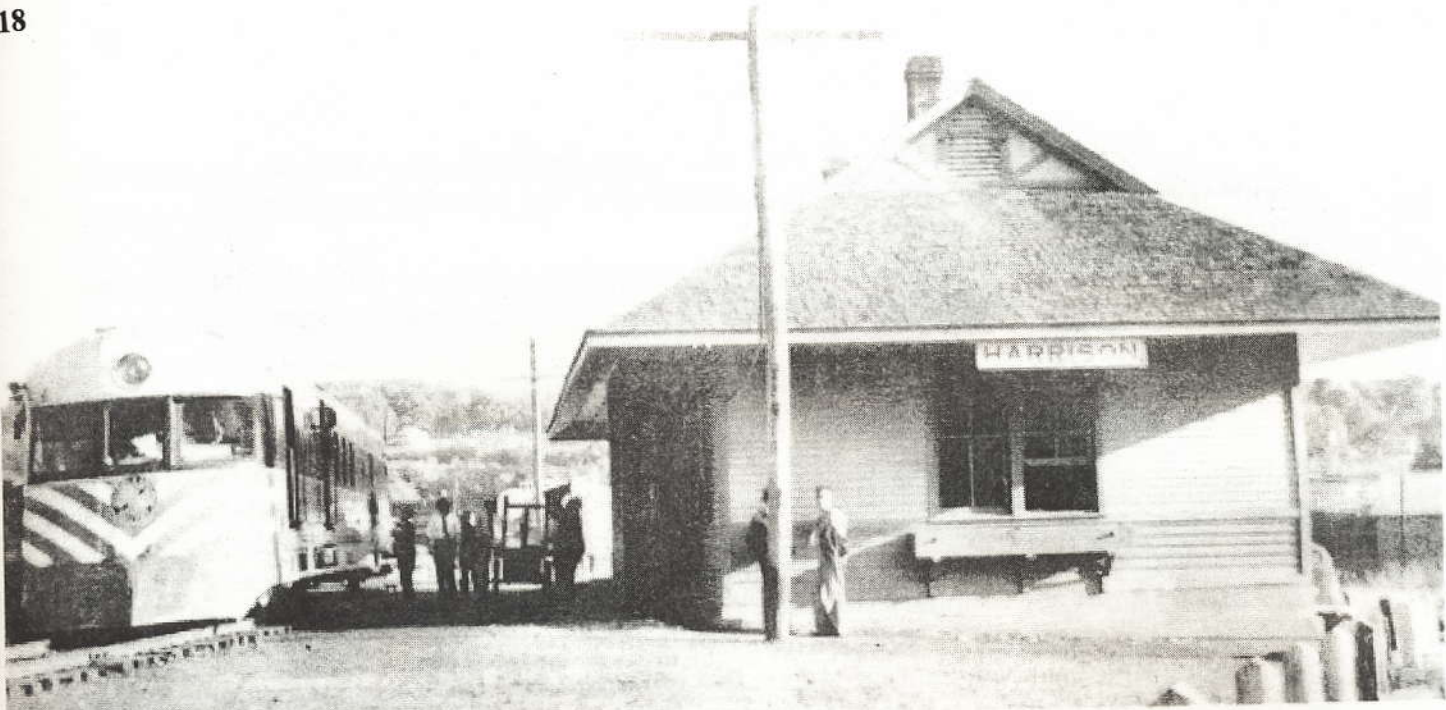
Missouri & Arkansas Diesel Motor Car with Train No. 705 loading baggage at the Harrison, Arkansas depot, March 8, 1944. (Ken Ziegenbein collection, photographer unknown)
