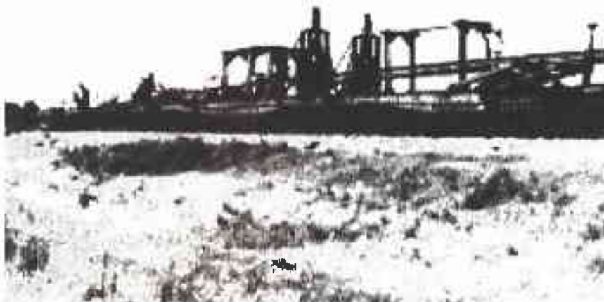
(32 Top) - A work train is loaded with lengths of welded rail and ready to roll down the main track to where a track gang waits to spike them in place; August 1974.
