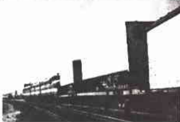
(20 Top) - In a new type of piggyback service, the Mo.P. had Thermo-King mechanical refrigeration units in some of its Truck-Rail trailers for handling perishable shipments. This one was at North Little Rock, Arkansas in 1961. (21 Bottom) - In an early piggyback shipment, a pair of Kansas City Southern trailers were riding a Trailer Train flat car toward St. Louis behind ALCO FA-2 No. 382. Photo at North Little Rock in 1955. (Gene Hull photos)
