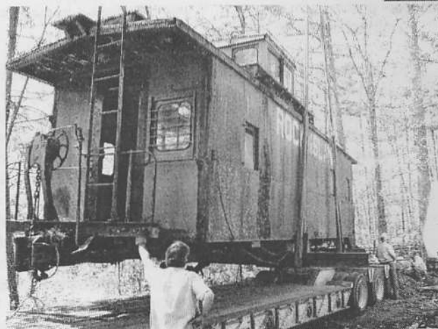
With incredible precision, the crew lowered it onto a low-boy trailer. Using chains, the caboose body was secured onto the trailer for transport.
