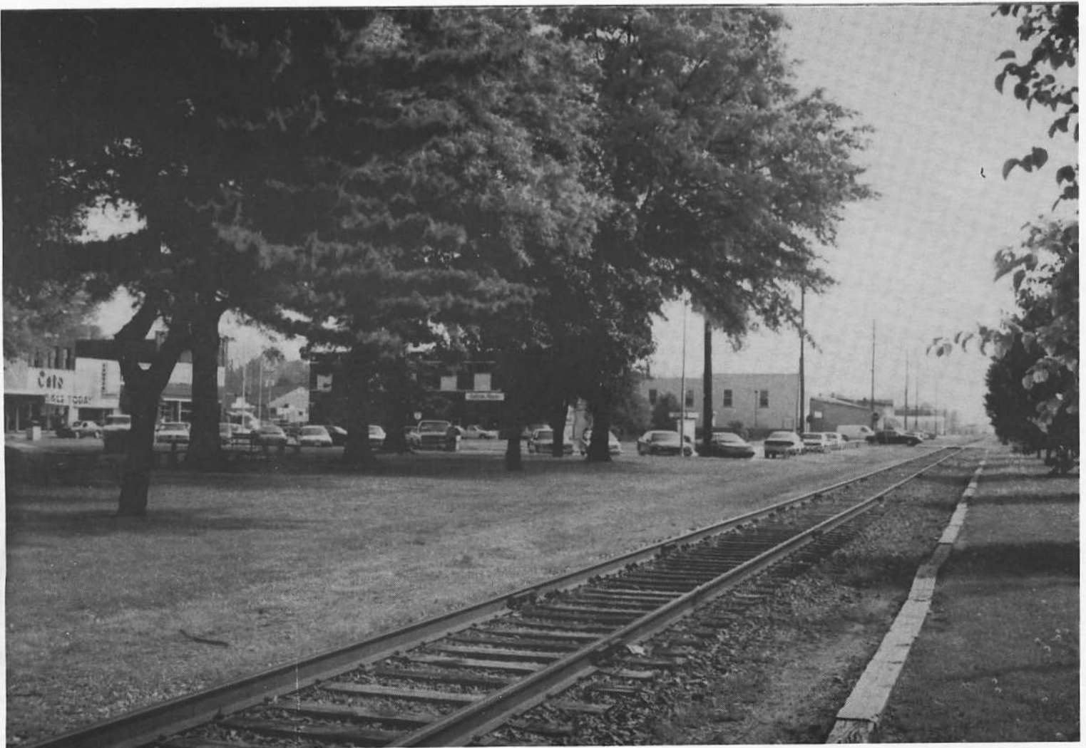
Looking east from the city park in downtown Sikeston, Missouri along the former Missouri Pacific tracks. The tracks only go a few more miles east, being taken up before reaching Charleston. (Ken Ziegenbein photo)
