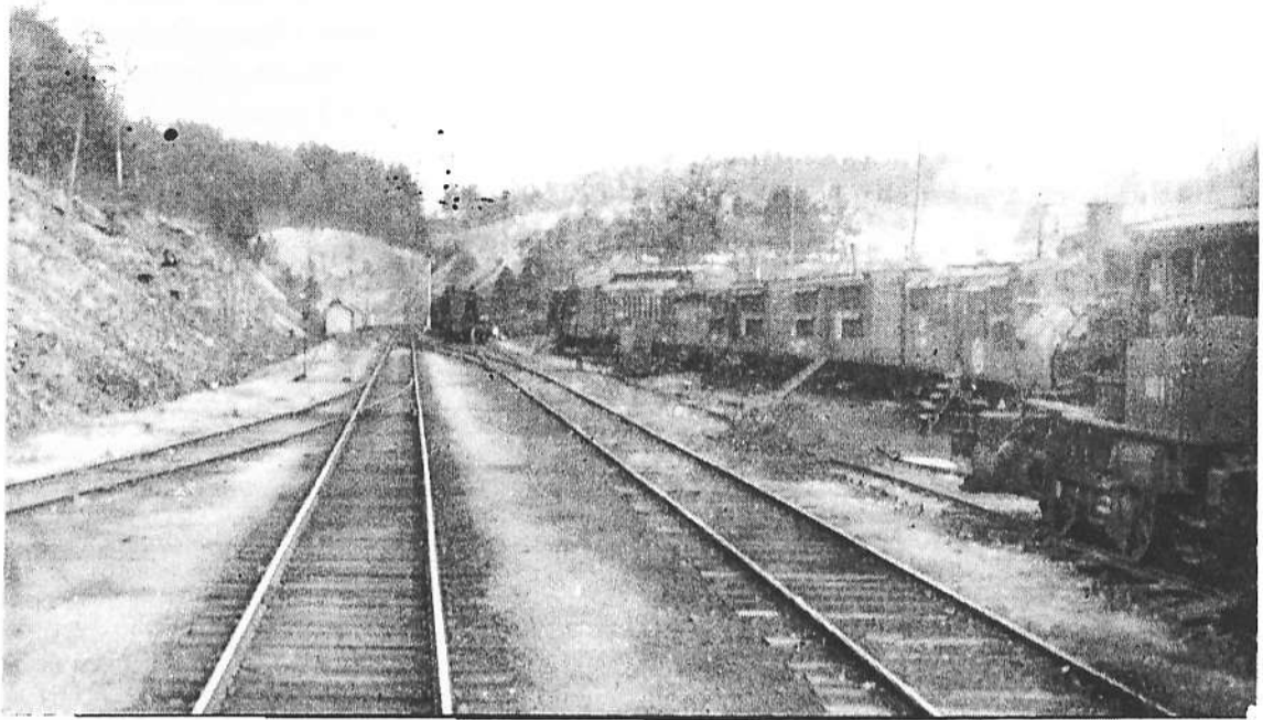
It is unfortunate indeed that this picture is so dim. It just about covers the most important features of Cricket. House track switch coming in on left (north). Main line and siding and several yard tracks with the little 0-4-0 sharp right and bridge gang strung up and down. The portal of the tunnel is hidden by the section tool house against the hillside to left. The semaphore signal is just to left of cars on down on an extension of the siding. You can barely see the raw hillside to the right where tons and tons of rock was dug out. That work was complete and this gang is putting in the last of the new steel bridges. (Picture by Barringer 1935. Collection of Bill Hoss)
