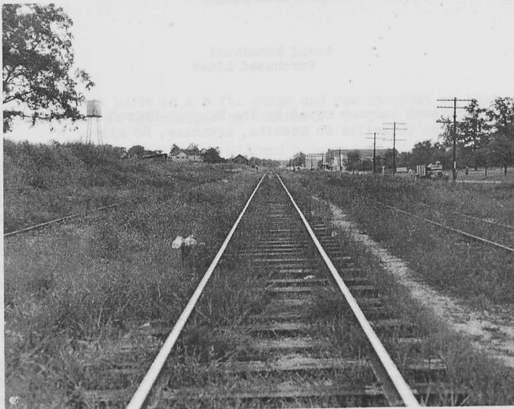
A Rock Island accident investigation photo taken at Hodge, Louisiana on September 9, 1942, between 3 and 4 p.m. looking south. They were investigating the September 6th death of a trespasser at a road crossing just north of the depot (seen just to left of center in the distance). (L. T. Walker collection)
