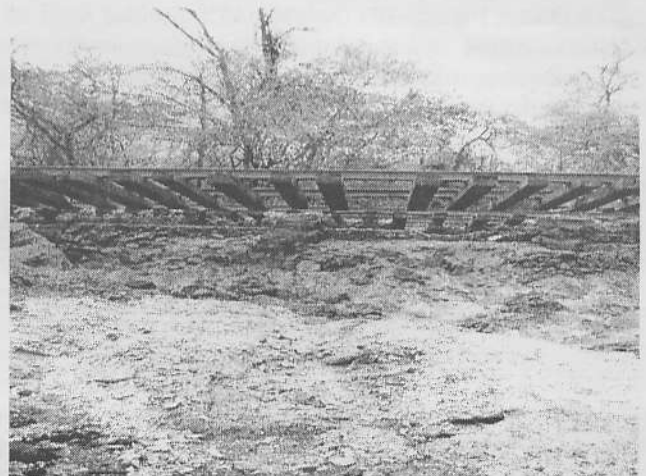
LEFT - Small trestle at milepost 364 and damage from massive flooding. RIGHT - A&M mainline dangling after washout at Winslow, Arkansas April 24, 2004. (Photos courtesy of Mike Sypult)
