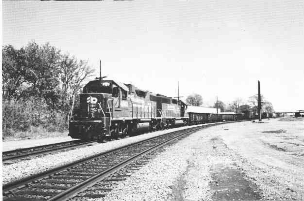
TOP - A view from the overpass showing various Southern Pacific (Cotton Belt) buildings in the yards at Pine Bluff soon to be demolished. The building to the left and the two next to the tracks are to be razed sometimes this year. The large building in the center is home to the Cotton Belt Rail Historical Society and Cotton Belt #819 and this building will probably be preserved. BOTTOM - SP 4863 and 7115 heads a Little Rock local out of Pine Bluff in April 1997. (Both photos by John C. Jones)
