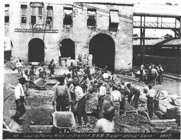
Laying paving bricks in front of P.R.R. freight office in Colon, Panama, 1907. (Courtesy National Archives, Clifton E. Hull collection)
