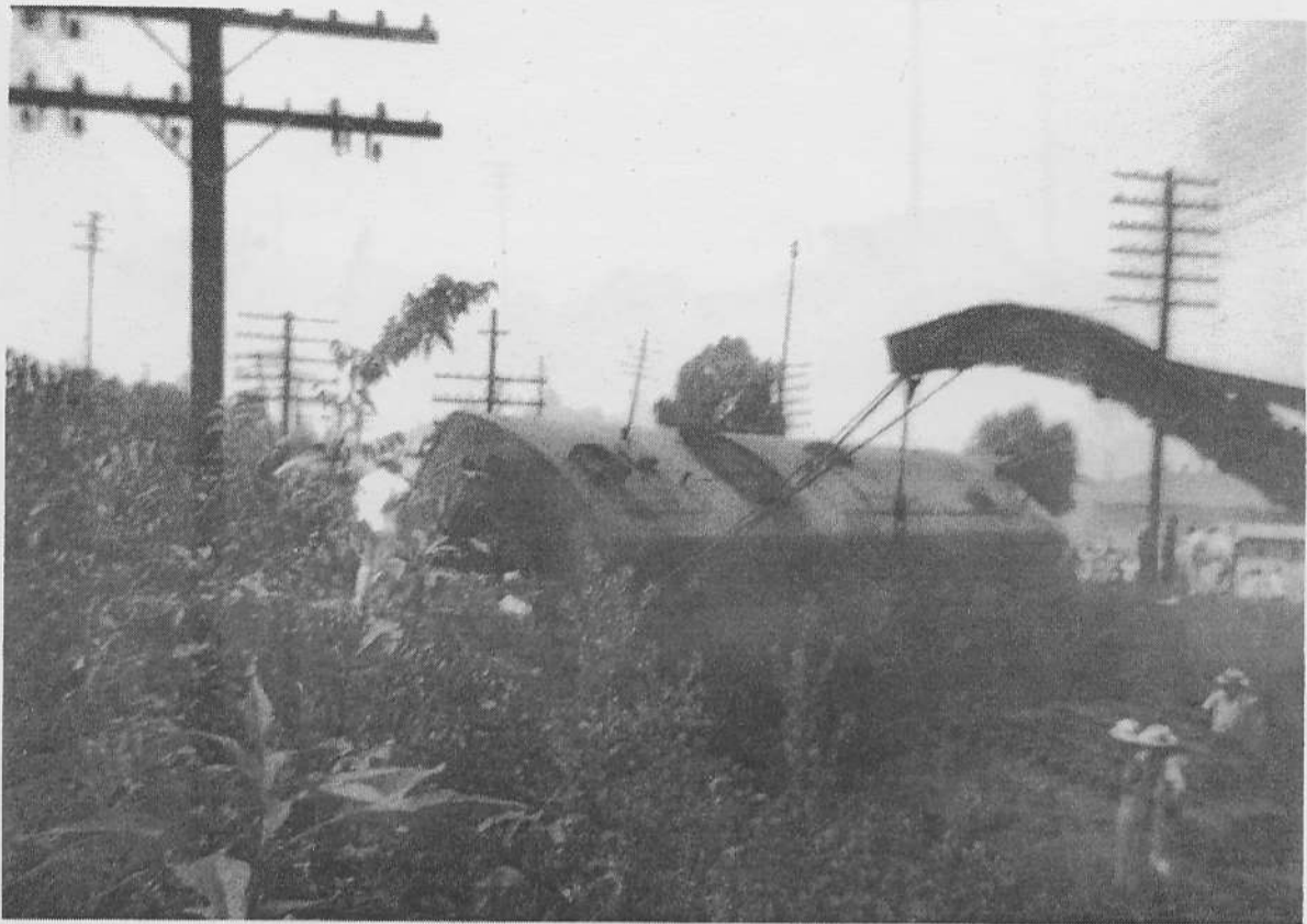
The T&P "big hook" from Texarkana has hold of the rear end of PA #8002A and is about to set it down on the track panels seen in the right foreground. (John A. Mills photo)
