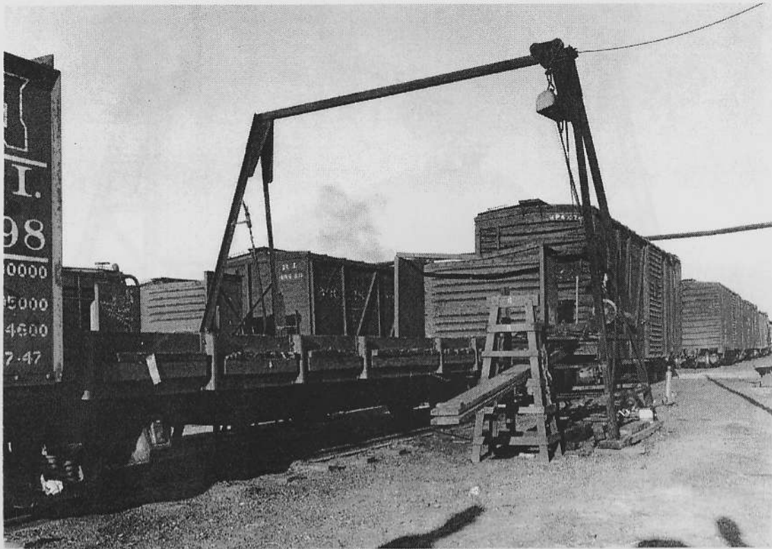
Rock Island accident investigation photo taken at Biddle Yard, Little Rock, sometime in the late 1940s. Shown is the "A" frame over rip track No. 6. They were investigation some accident at the yard. ( L. T. Walker collection )
