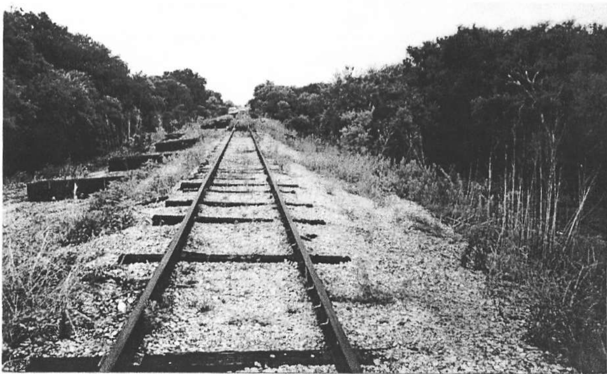
Example of rehabilitation work. At MP 98.6 a wooden trestle is being replaced. View toward the south, July 4, 1998.
