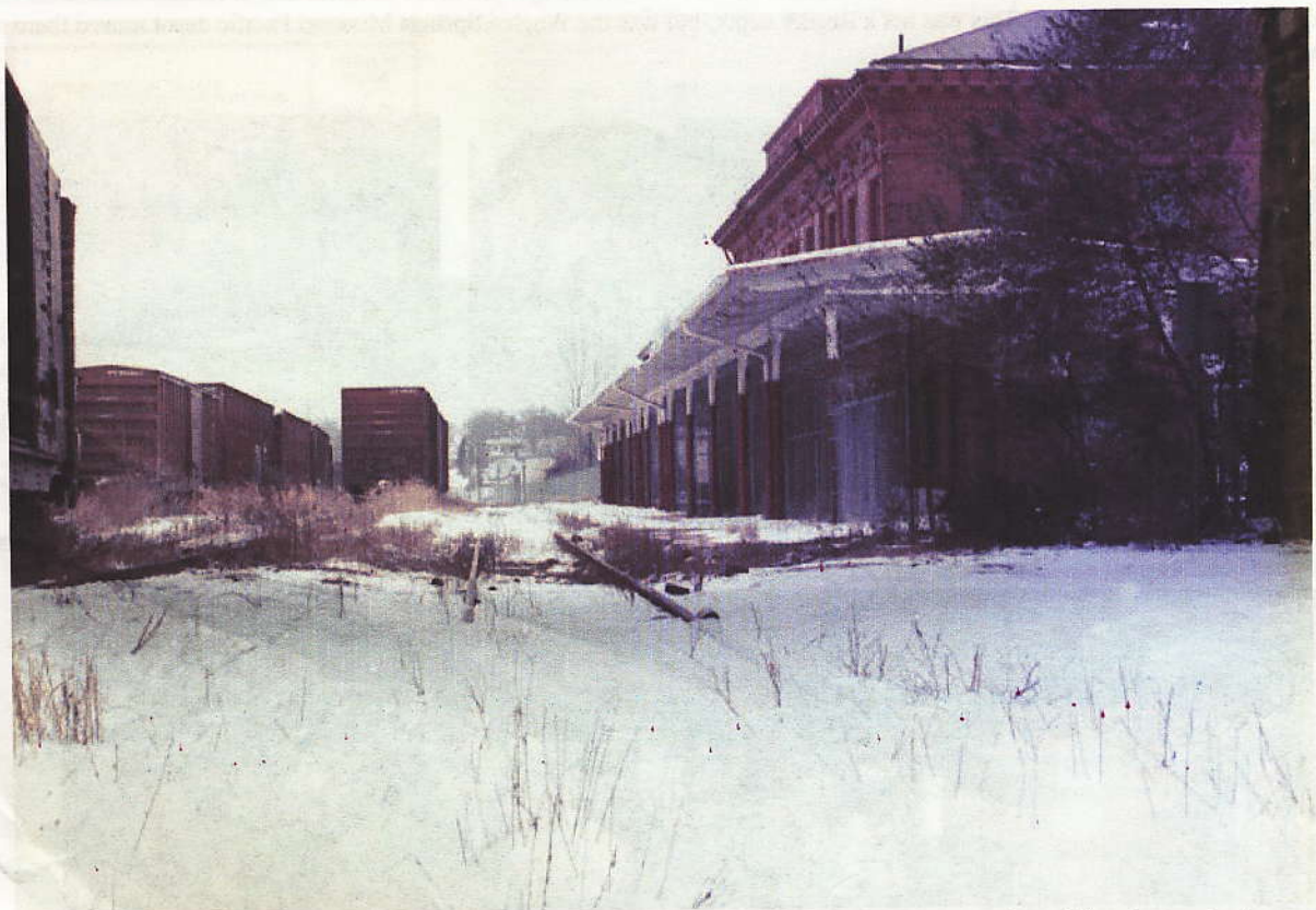
Rock Island's Choctaw Route depot in Little Rock had been vacant for many years when this wintry photo was taken in February, 1985. This passenger station has been preserved and will be part of the Clinton Presidential Library - the old Choctaw Freight Depot that was across the tracks to the left was demolished in November 2001 for the library. (Ken Ziegenbein photo)
