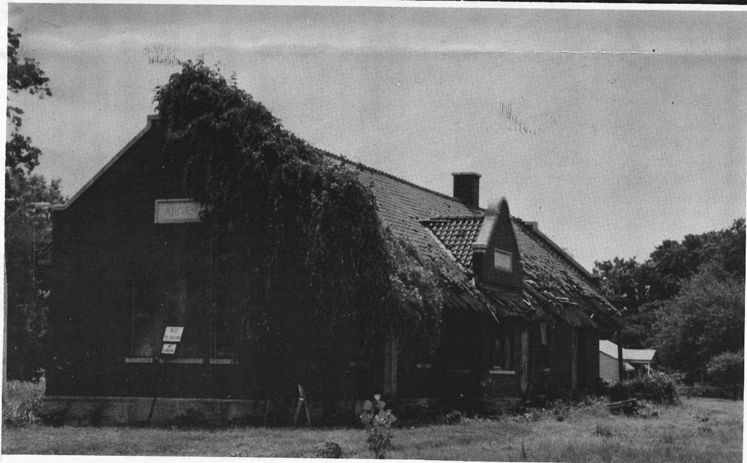
On July 23, 1994, a few from the Arkanssa Railroad Club headed by John Hodkin, Jr, cleared grass and trees from the Argenta Rock Island depot in North Little Rock. Here is the before (Above) and after (Below) look of the depot.
