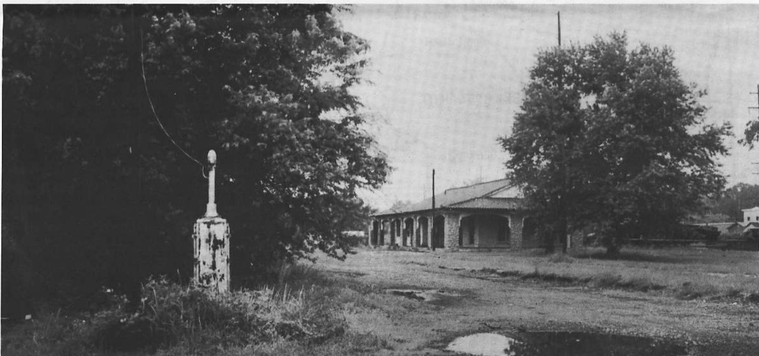
TOP -Booneville's old Rock Island depot was still in relatively good shape on May 13, 1994. It is owned by the junk yard owners just to the west of it. BOTTOM - The old signal box was also still in place in May 1994. The tracks ran just to the left of the station. Tracks were taken up in the early 1980s. (Ken Ziegenbein photos)
