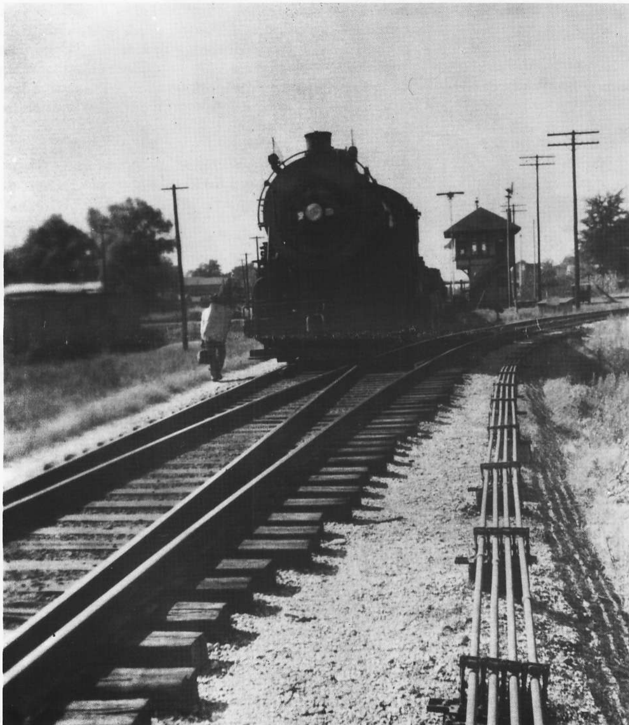
A Rock Island Extra southbound freight train pulling by the Fordyce Tower in Fordyce, Arkansas during the early 1940s. The pipes on rollers were what moved switches, derails and signals. The track bearing to the right connected with the Cotton Belt toward Pine Bluff. (P. B. Wooldridge photo)
