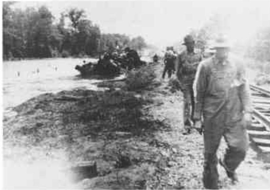
A Kansas City Southern wreck of a caboose hop caused by a washout at Bridge C-453 (Flat Creek) just south of Winthrop, Arkansas circa 1943. Brakeman Frank Huckabee of Texarkana was killed in this wreck (by drowning). The train had just dropped off 15 Pullmans full of Army WAACS to the Missouri Pacific at Texarkana and was heading for DeQueen on the KCS. (Philip L. Moseley photo)
