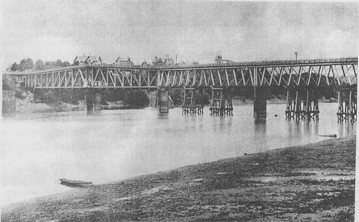
This is a view of the original Baring Cross bridge for the Cairo & Fulton railroad early in 1890. Note railing along the top of the wood trusses. (Gene Hull collection)
